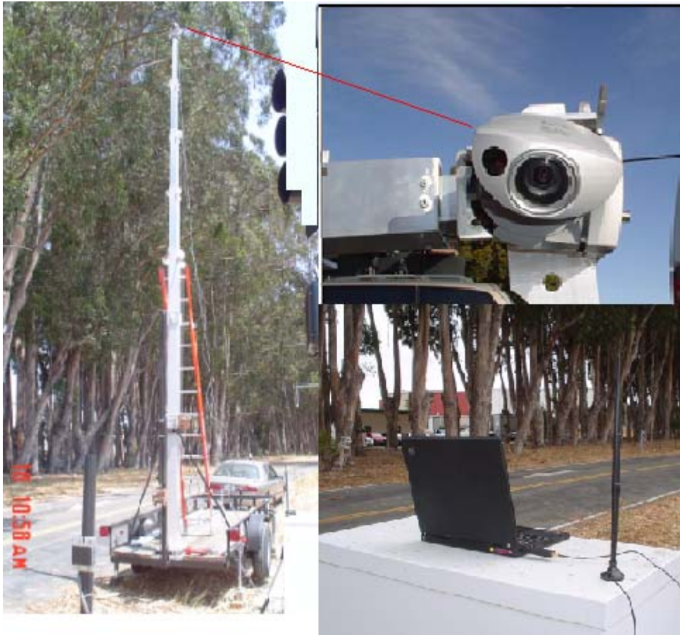
Figure 2. Left: Mobile retractable pole; Upper right: PTZ camera on top for looking at the loop and for vehicle tracking to obtain baseline data; Lower right: video computer also running IEEE 802.11b wireless communication using USB port.
